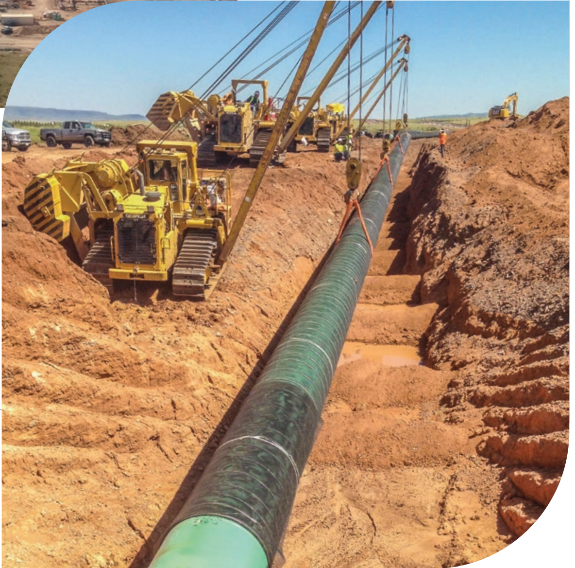
Waha-Presidio gas duct
