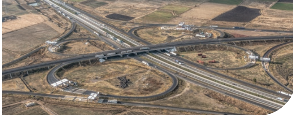
North Arc Beltway
