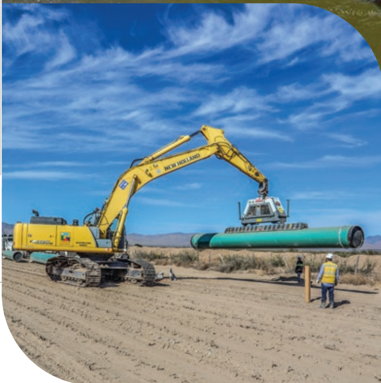
Samalayuca-Sásabe Gas Pipeline
