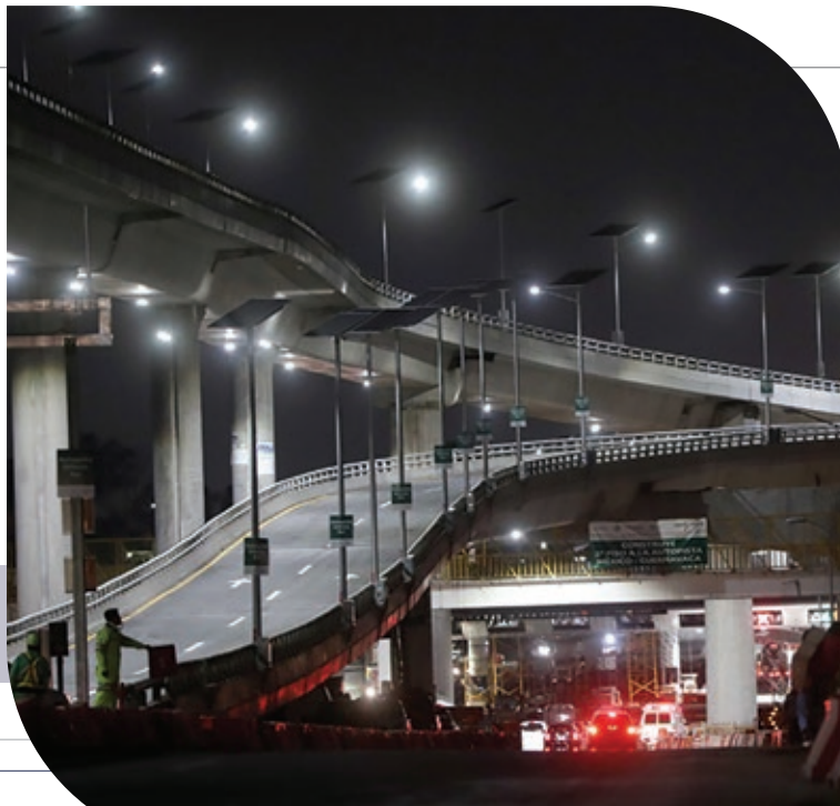
Southern Urban Toll Road
