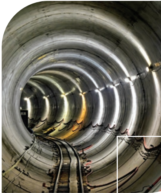
Emissor Oriente Tunnel
