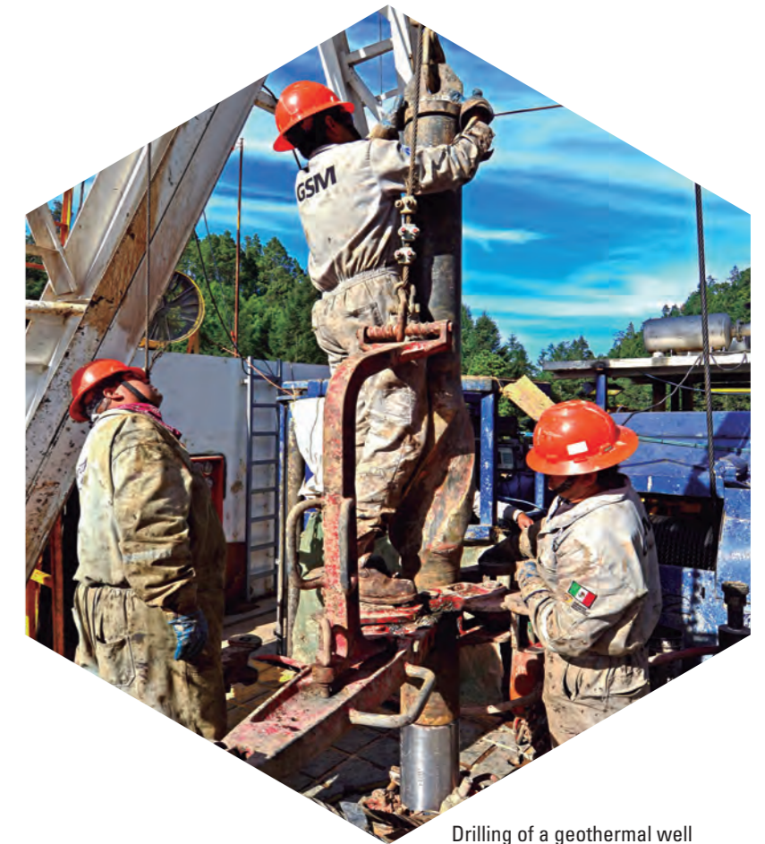
Drilling of a geothermal well
